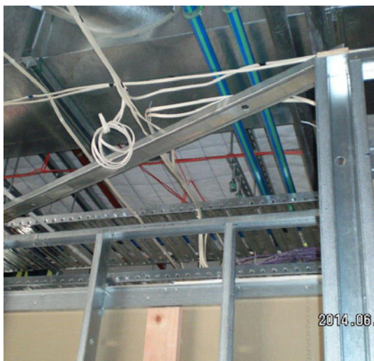
Figure 74: Horizontal bracing.
