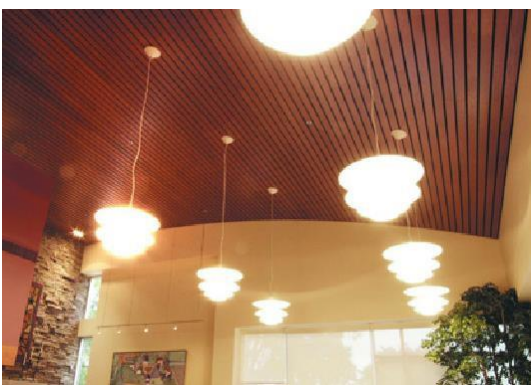
Figure 17: Proprietary linear ceiling system.
