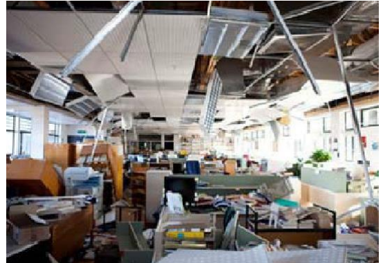
Figure 82: Damage to ceiling tile from an unrestrained fire protection system.
